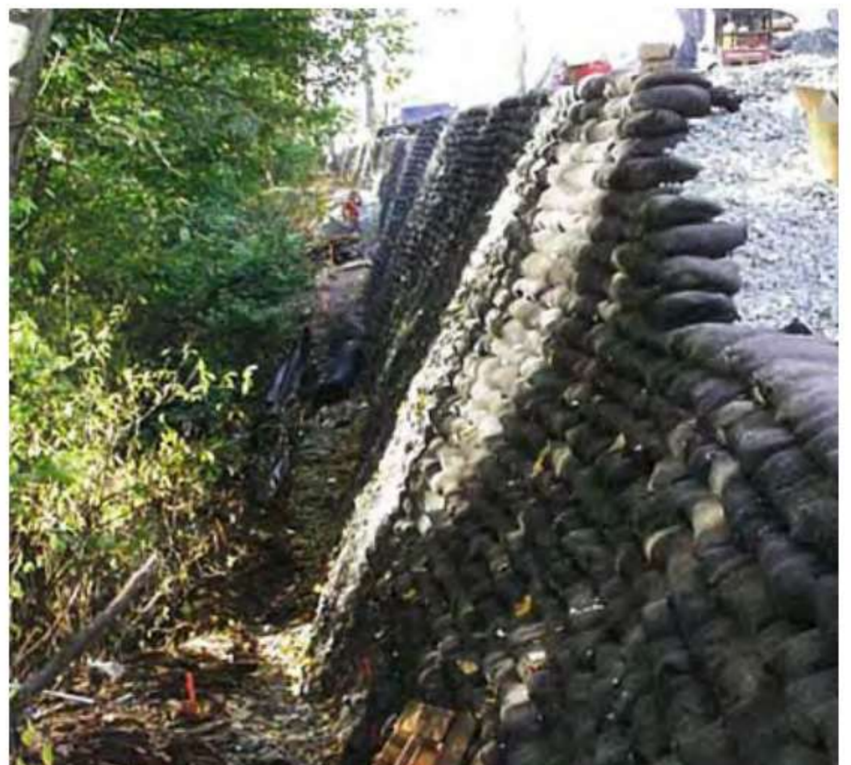
Deltalok during construction
