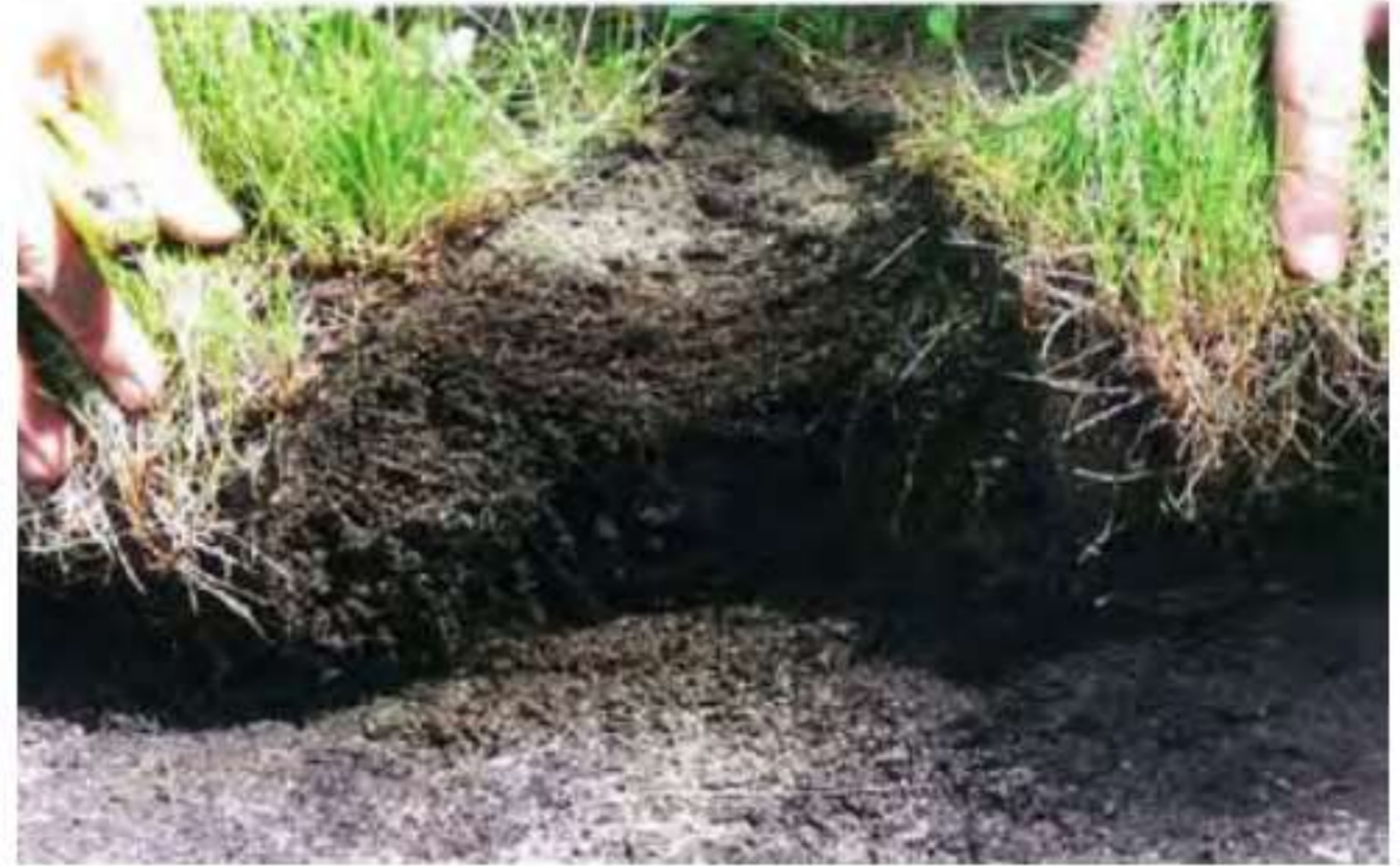
Deltalok root penetration exposed in a cut ecology bag
