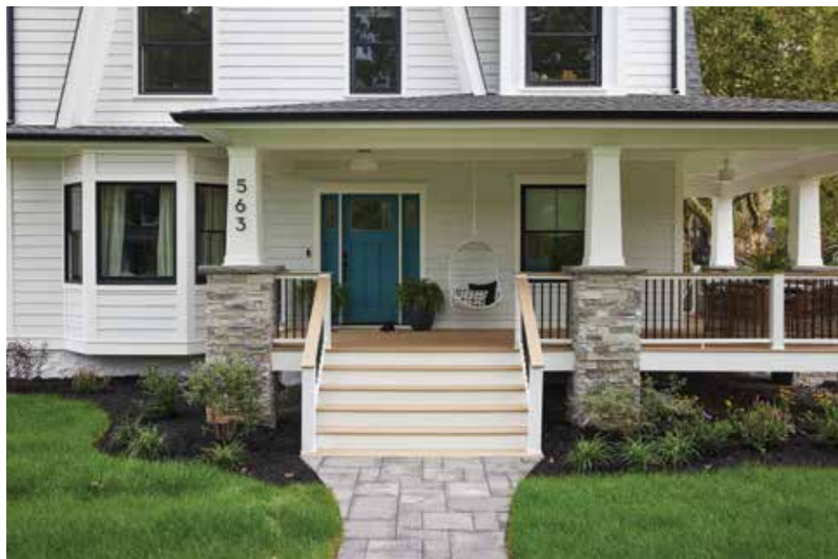
Weathered Teak® Porch + AZEK® White Trim Boards as Fascia and Risers + AZEK White Tapered Column Wraps
